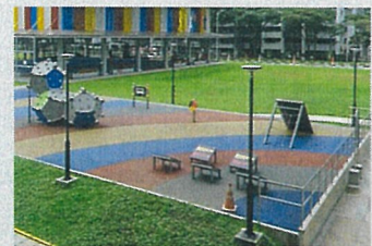
Construction of Playground near Blk(s) 128 Lorong 1 Toa Payoh
