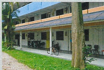
Construction of Fixed Awning at Ground Floor Corridor of Blk(s) 104 Lorong 1 Toa Payoh
