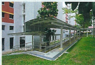
Construction of Shelter over Existing BFA Ramp near Blk(s) 449 Sin Ming Avenue
