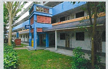
Construction of Fixed Awning at Ground Floor Corridor of Blk(s) 106 Lorong 1 Toa Payoh
