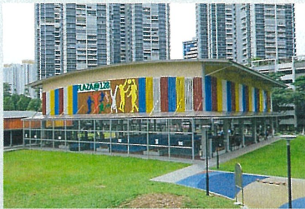
Construction of PLAZA@128
