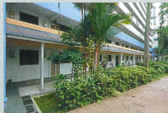
Construction of Fixed Awning at Ground Floor Corridor of Blk(s) 105 Lorong 1 Toa Payoh
