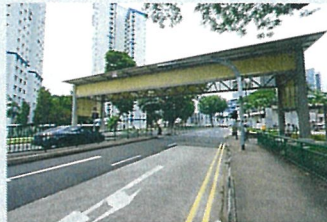
Construction of High and Low covered linkway from Blk(s) 138 Lorong 1A Toa Payoh MSCP to Covered Plaza at State Land near Blk(s) 127 Lorong 1 Toa Payoh
