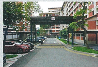
Proposed New Covered High and Low Linkway Connecting Blk(s) 215 and 216 Bishan with New BFA Ramp
